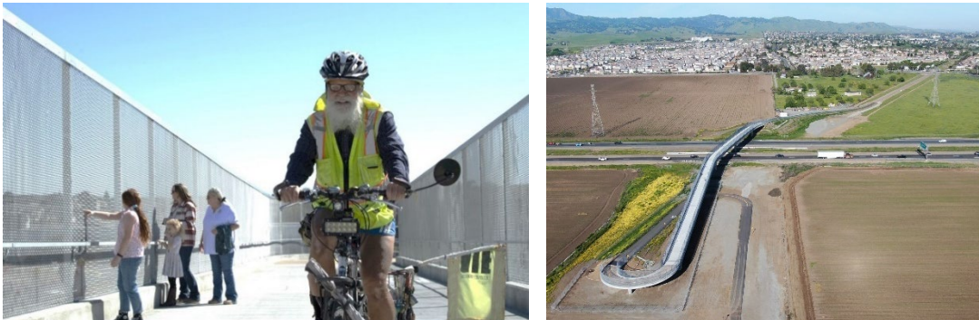
Mokelumne Trail Bicycle/Pedestrian Overcrossing of State Route 4. Contra Costa Transportation Authority Photo
