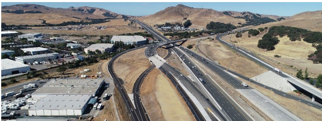
First RM3-funded construction package for the I-80/I-680/SR-12 interchange in Fairfield. Caltrans photo
