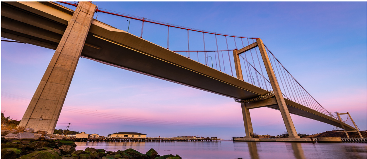
View from below of the Alfred Zampa Memorial span of the Carquinez Bridge. Photo: © Chris LaBasco Photography, Getty Images/iStock.
