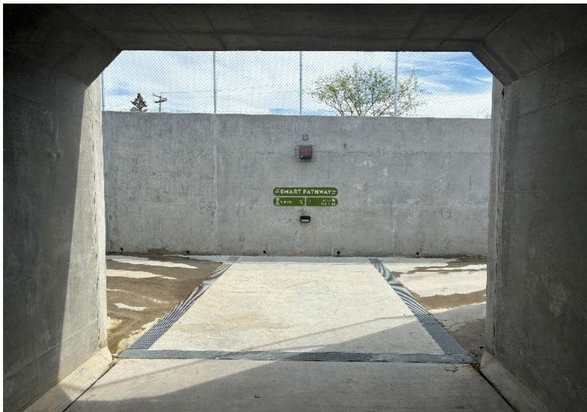
SMART Windsor High School Undercrossing. Photo: SMART
