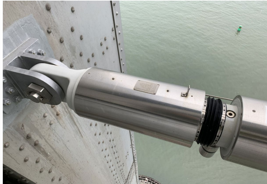
San Francisco-Oakland Bay Bridge Replace Seismic Dampers:
