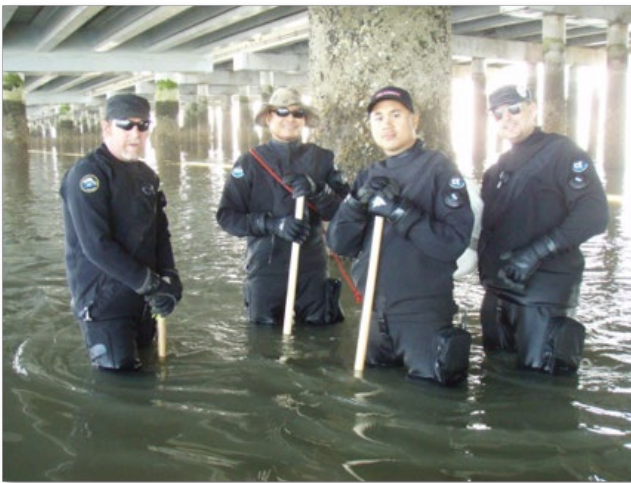
Figure 1-C: Bridge underwater inspection
