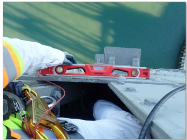
Figure 1-D: Physically measuring flatness
