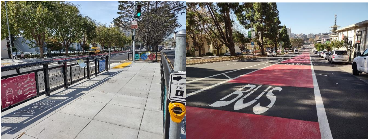
Completed Geary Rapid Station and red colored lane (source: SFMTA)
