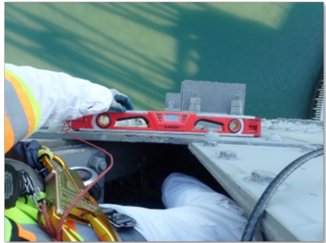
Figure 1-D: Physically measuring flatness
